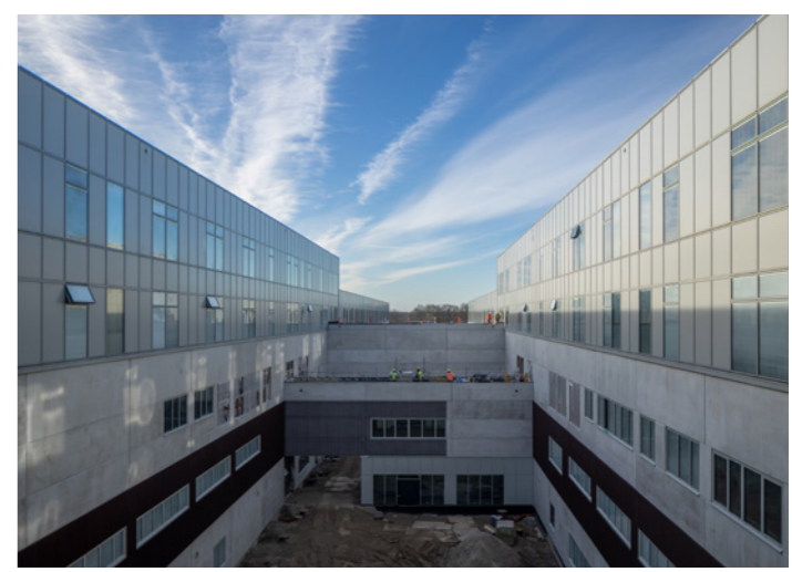
Construction site photo
