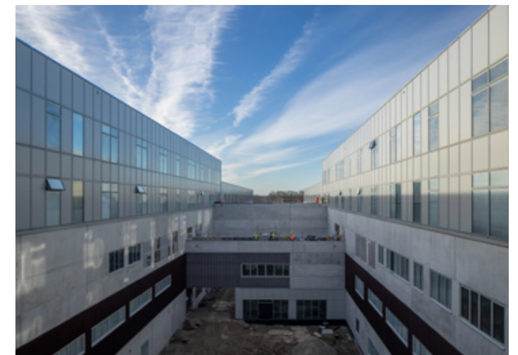
Construction site photo
