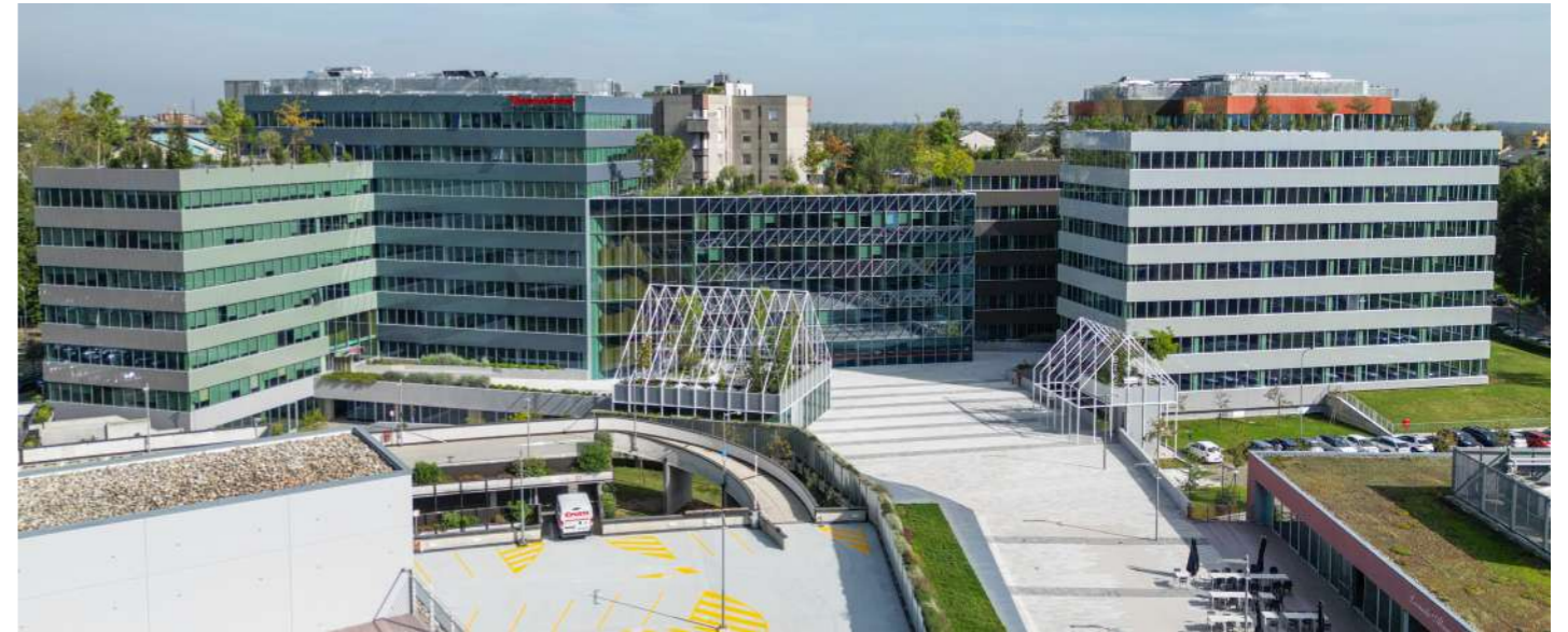
Project Management per Segreen Buildings, Segrate, Italia
