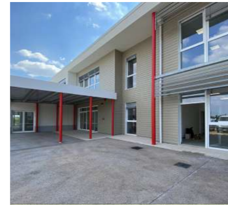
EXTENSION OF PRIMARY SCHOOL "S. PELICO" Lugagnano di Sona, 2020 € 2.5 mln - 2.100 smq, Final and executive design, CSP, AR -ST - MEP
