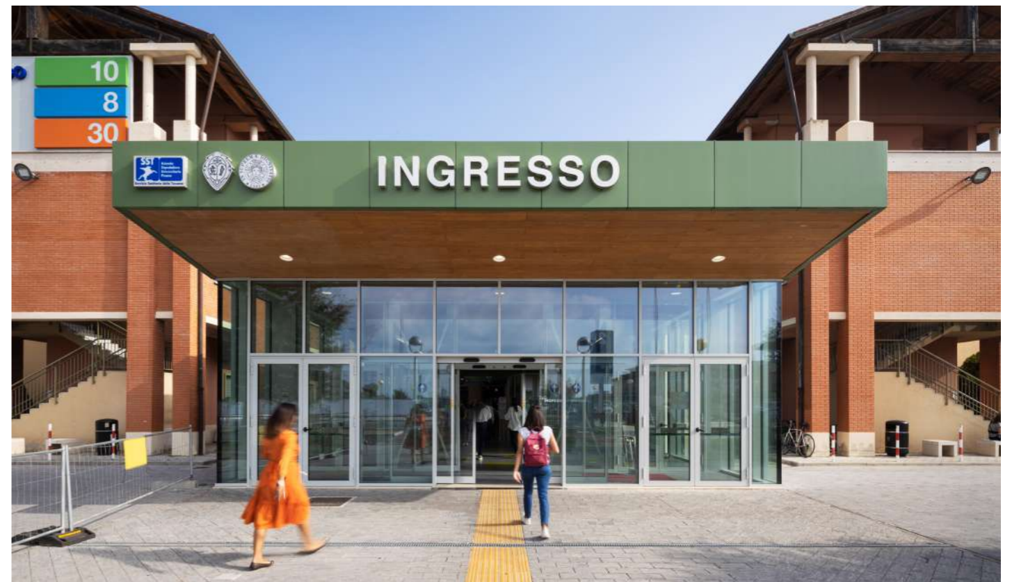
Cisanello Hospital Complex Expansion, Pisa, Italy
