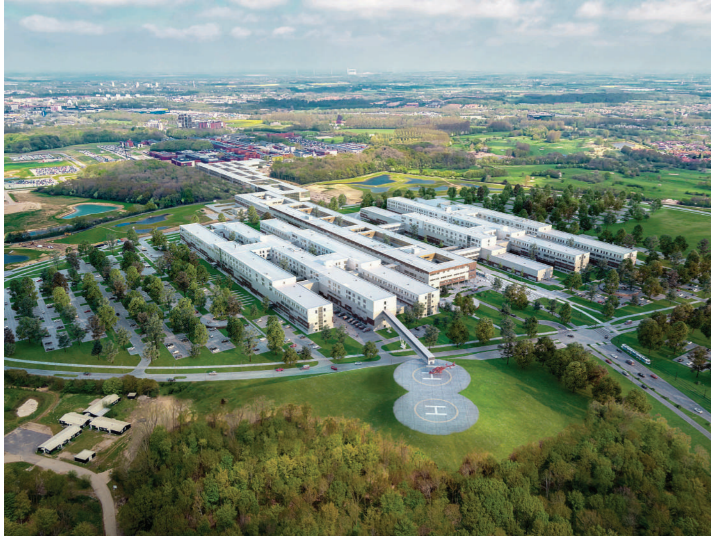
Nyt OUH University Hospital, Odense, Denmark
