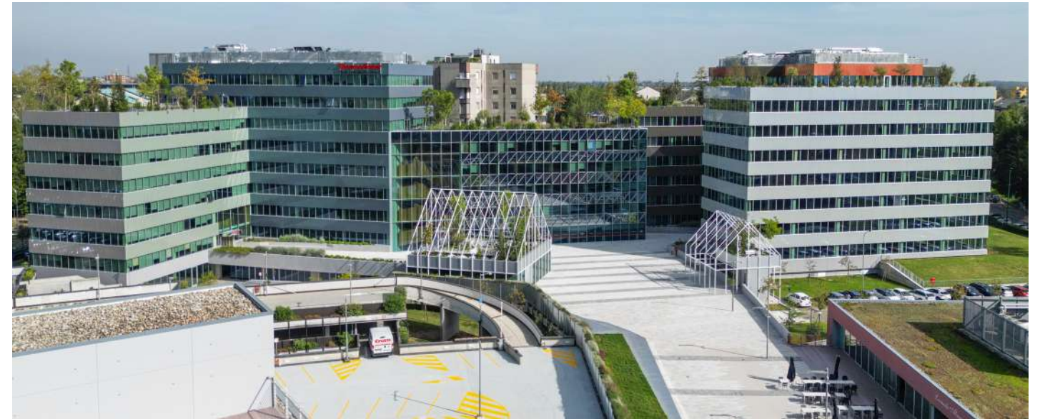
Project Management per Segreen Buildings, Segrate, Italia
