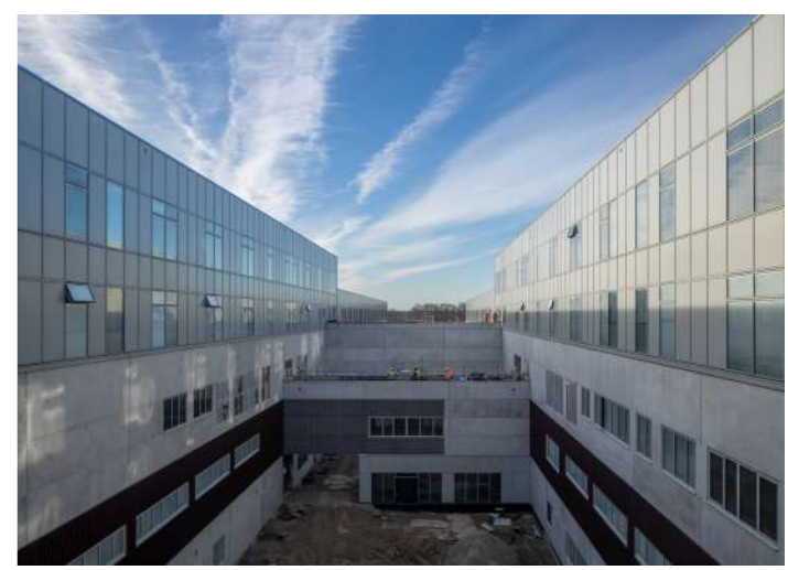
Construction site photo
