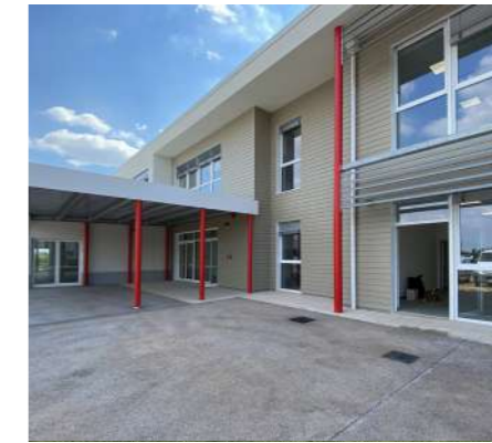
EXTENSION OF PRIMARY SCHOOL "S. PELICO" Lugagnano di Sona, 2020 € 2.5 mln - 2.100 smq, Final and executive design, CSP, AR -ST - MEP
